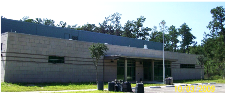
Tulane National Primate Research Center Quarantine Facility ($10 million)
